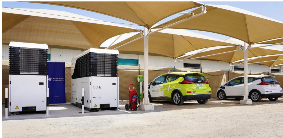
EV Charging UAE • Al Shandi
