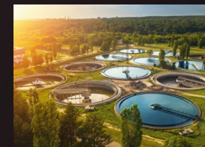
Sewage treatment plants
